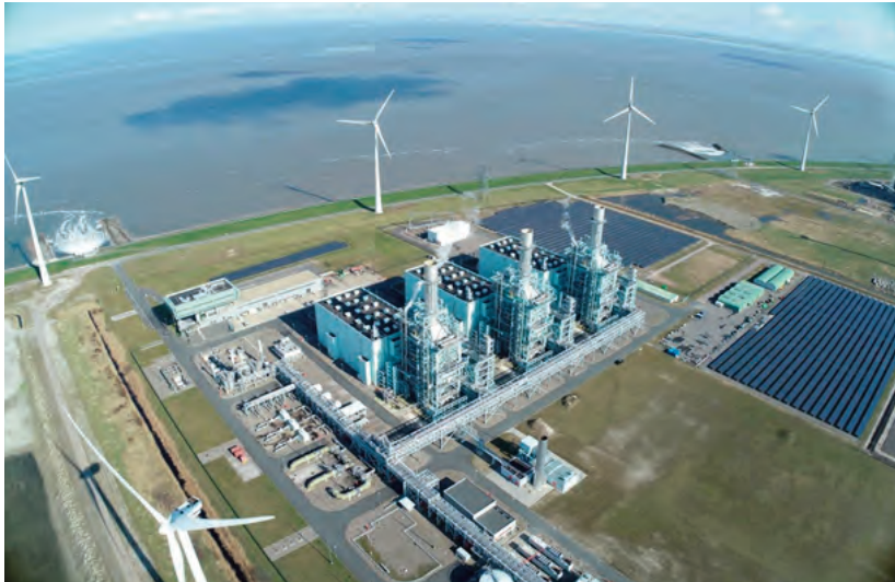
Abbildung 4.13: Magnum Hydrogen Thermal Power Plant 24
