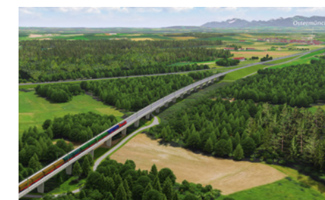
Feeder Line North of the Brenner Base Tunnel, GER, AUT
