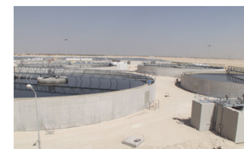
Sulaibiya Wastewater Treatment and Reclamation Plant, KUW
