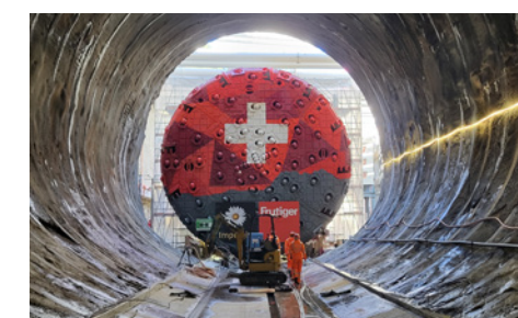
Gotthard Road Tunnel, SUI
