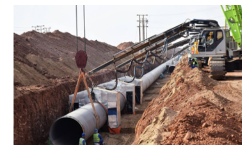
Ras Al Khair-Riyadh Water Transmission System, KSA
